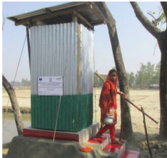
Figure 5: (left) Flooded pit latrine in Rangpur, Bangladesh in 2019. (right) Elevated latrine in Satkhira, Bangladesh in 2021. (Image source: UNICEF 57 )
